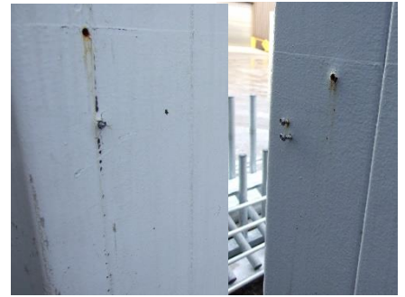
Bolt holes inc screws and bolts attached
