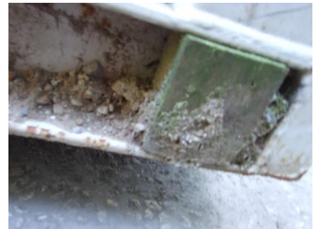
Concrete splashes on base of unit
