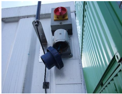
Damaged Commando Socket
