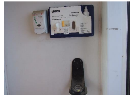
Customer equipment left in unit – removal, repair and holes to fill
