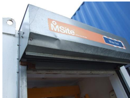
Dent to Roller Shutter
