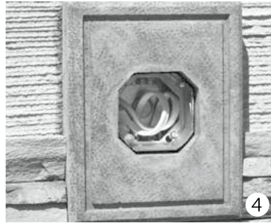
Complete placement of Cultured Stone veneer or other exterior material around Electrical Box Stone.
