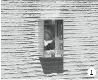
Attach UL-listed extension box to pre-wired and mounted electrical box.
