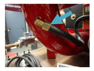
Tighten the nut as tight and you can with your fingers and then lightly tighten with the crescent wrench, pliers, or 13mm wrench. Thread should almost fit completely on the elbow.
