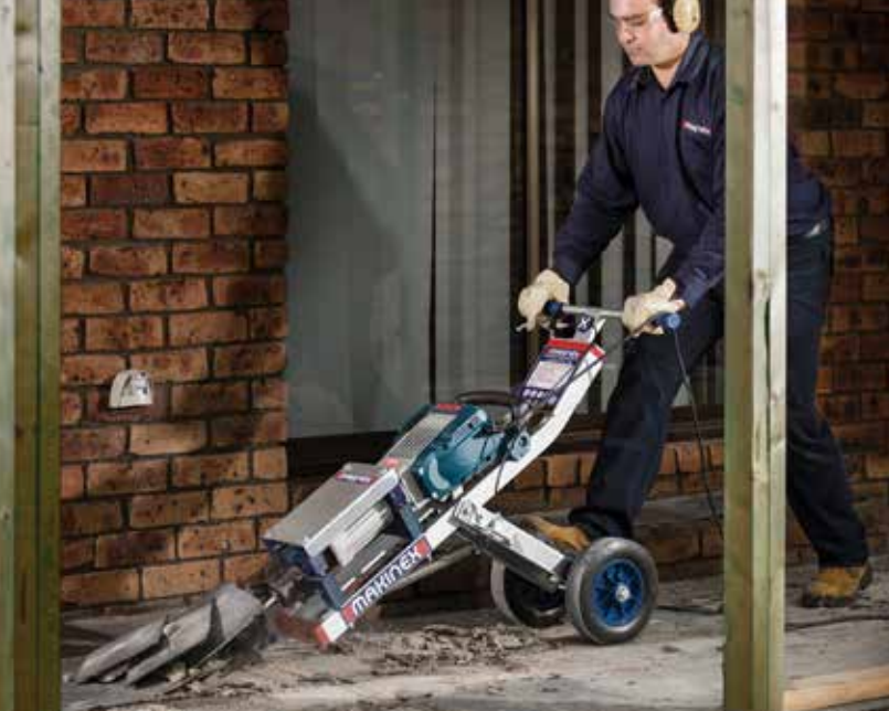
The JHT suits most 16kg jackhammers.
