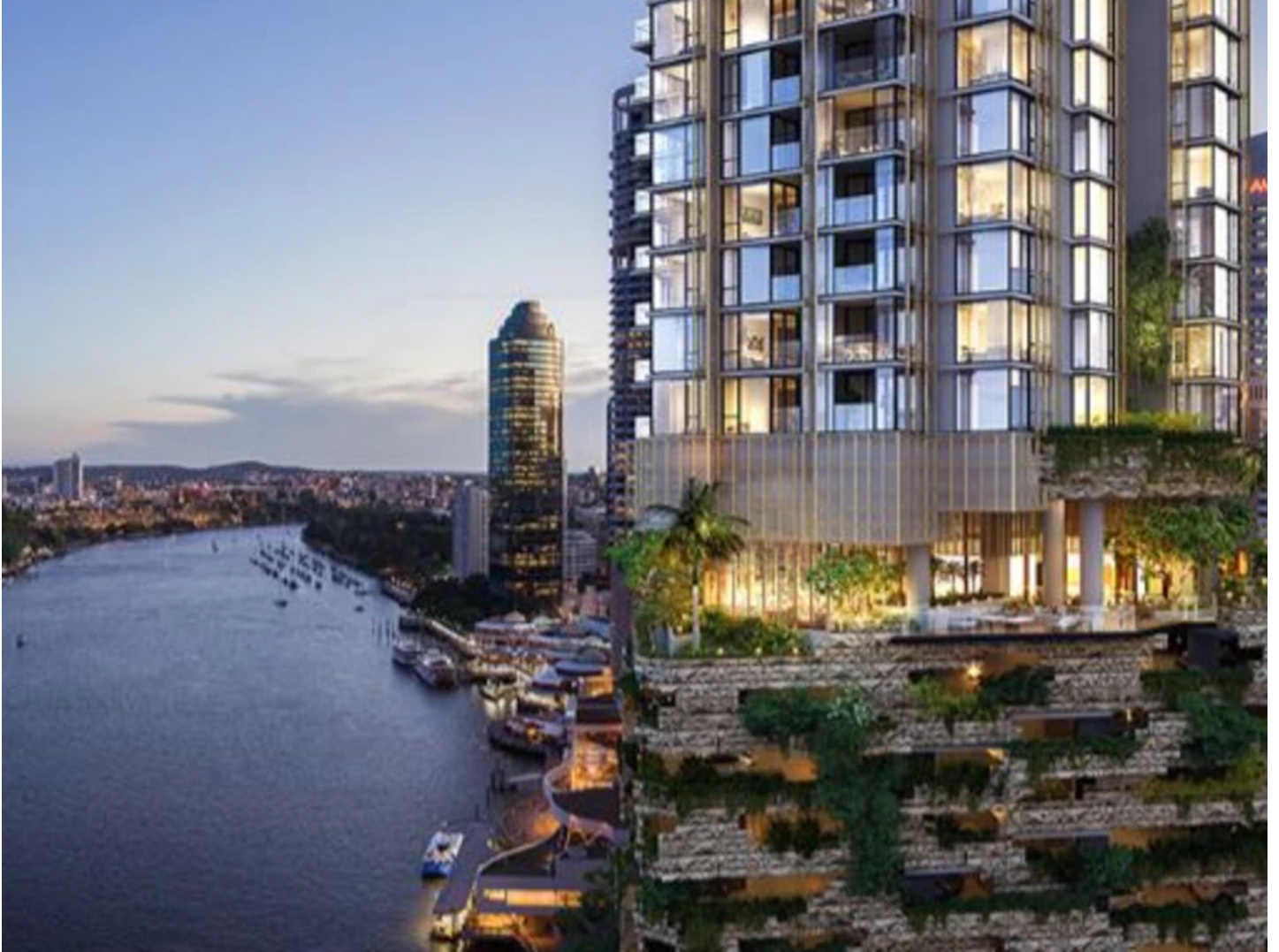
433 Queen St is estimated to cost $375 million to construct and will be another skyscraper towering over the Brisbane river. Picture: Supplied
