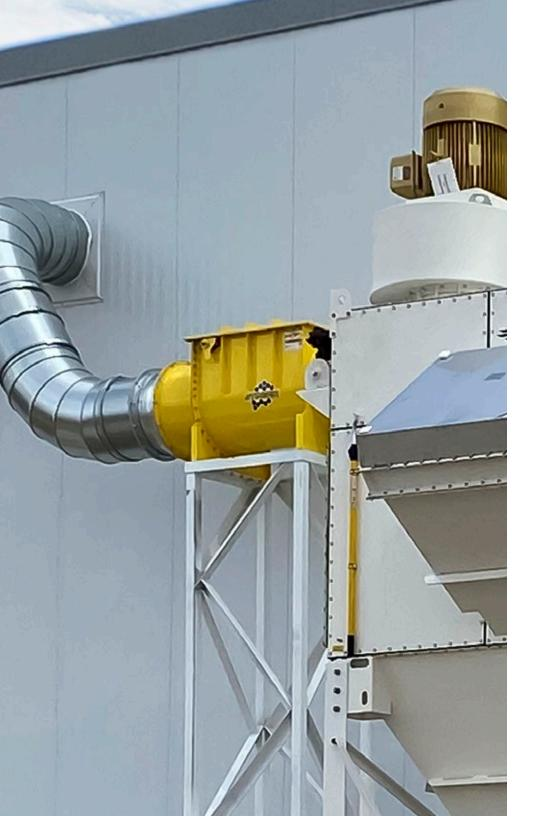
If an explosion vent is feasible, you will then determine what size and how many are required, the location where the dust collector will be placed and how much explosion vent ducting (if any) will be required. The inlet and possibly the outlet ductwork must also be protected against the possibility of an explosion as determined by a risk assessment.
