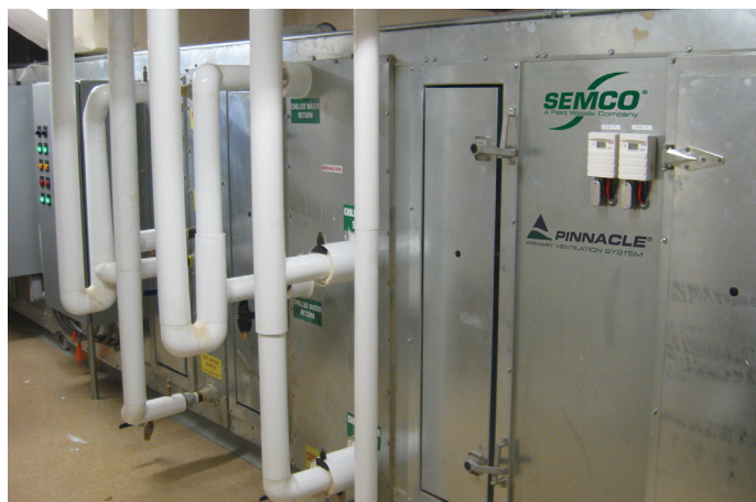
Customized SEMCO Pinnacle® Primary Ventilation Unit.
