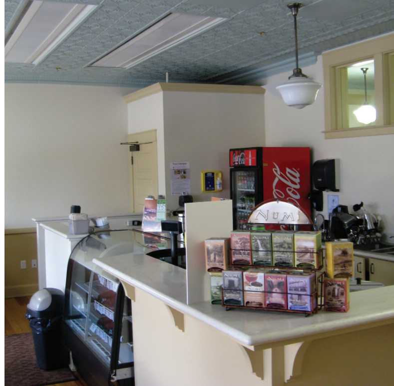
Chilled beams conditioning the Peabody Perks Coffee Shop.
