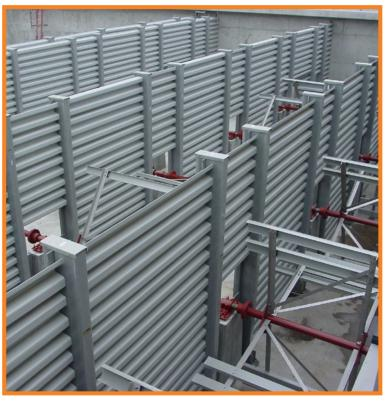
Flocculation Baffle Walls using Enduro Baffle D
