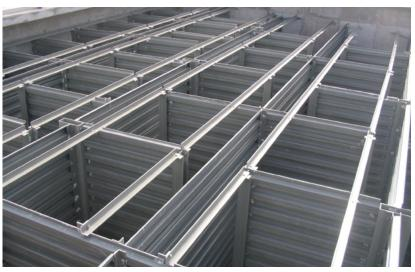
Enduro "D" & "H" baffle wall systems with top-braced FRP columns Flocculation and Sedimentation Basin
