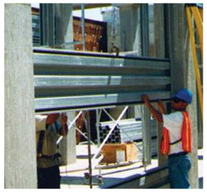
"H" series baffle panels are stacked from basin bottom to top and do not require fastening to supports.
