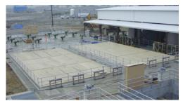
XL6 beam supported covers with access hatches 53'x 60' Pre-treatment Tank Complex
