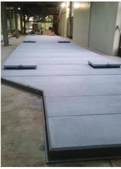
XL6 clear span tank cover system with angle cut panels and access hatches over filtrate storage tanks
