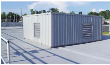
Tuff Span removable enclosure with FRP panels, beams and louvers over floating aerator. Beam-supported cover - Aeration Basin
