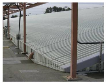
Tuff Span walk-in tank cover system with FRP translucent panels, beams, platforms and doors. Left photo shows the inside and right photo shows the outside. Aeration Basin
