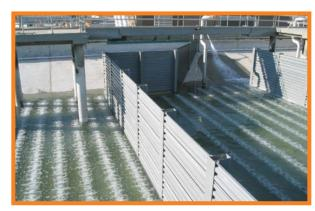
Enduro FRP SlideGuide "H" baffle series in aeration basin
