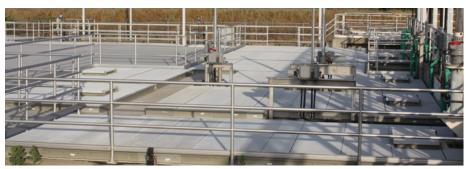
XL6 clear span tank cover system with access hatches UV Disinfection Process
