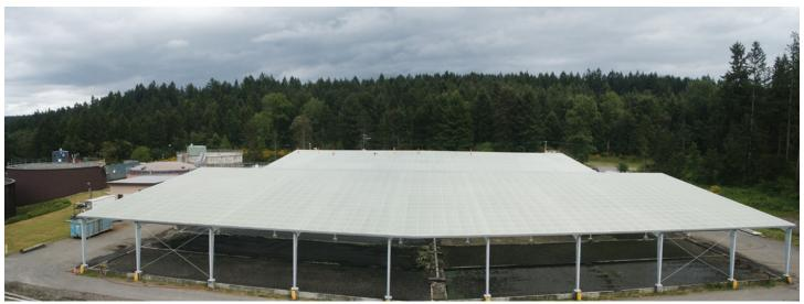
Tuff Span roof cover system Sludge Drying Bed
