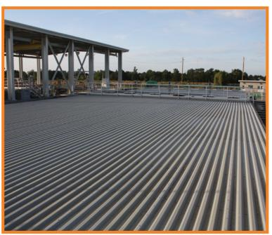
Tuff Span low-profile tank cover system with FRP beams **UV Disinfection Process**
