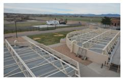
XL3 FRP Clarifier Tank Covers replacing Metallic Covers Supported by External Truss Support System
