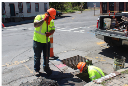
Cleaning out catch basins in Catskill
