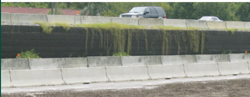
US-19, Florida – Over 100,000 square feet of Tensor Temporary retaining wall was used on the US-19 widening and reconstruction project in Clearwater, FL for FDOT.
