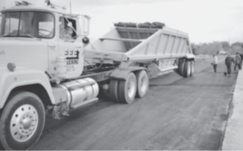
Image 8 Dumping aggregate fill on top of Tensar® Geogrid over competent subgrade.
