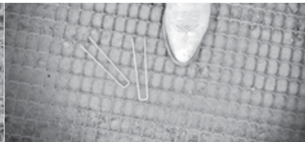
Image 7b Staples for anchoring BX Geogrid (optional).
