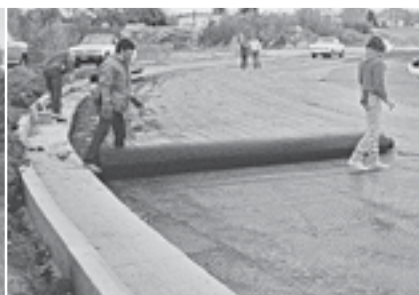
Image 5 Placing Geogrid to accommodate curves.
