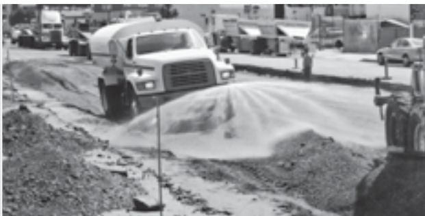
Image 10 Moistening the fill before compaction.
