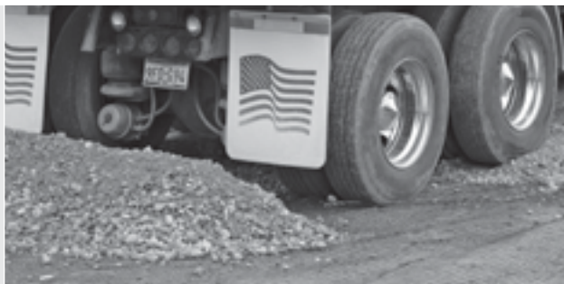
Image 12 Geogrid can be trafficked directly by rubber-tired equipment.
