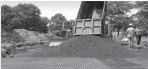
Image 9a End dumping aggregate fill on top of Tensar Geogrid over soft subgrade.
