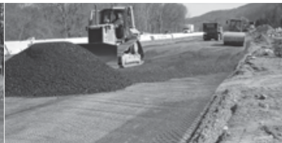
Image 9b Spreading aggregate fill over Tensar Geogrid.
