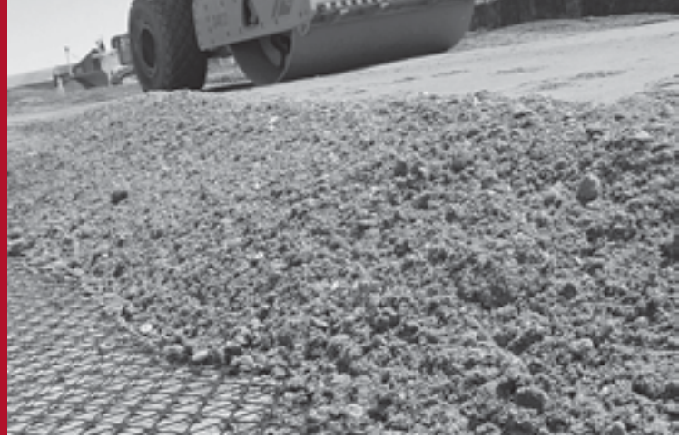
Image 11 Compacting the aggregate fill.
