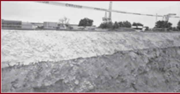
Image 13 A backhoe excavation through Tensar Geogrid.
