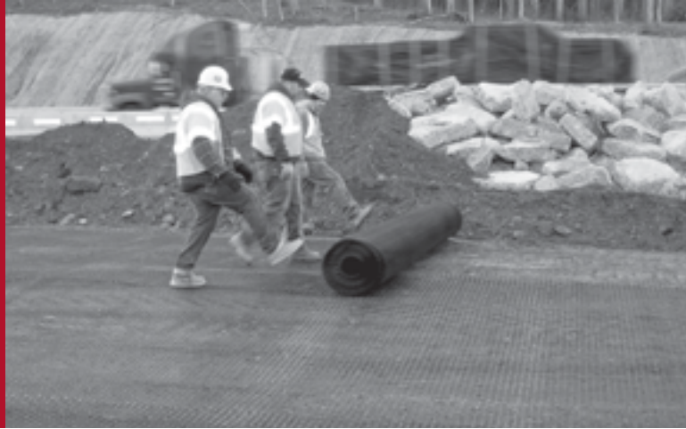
Image 3 Rolling out Tensor Geogrid.
