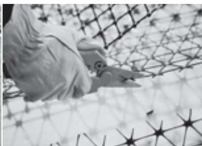
Image 6 Cutting Tensar TriAx® Geogrid is easily achieved.
