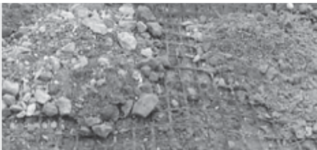
Image 7a Anchoring geogrid with piles of aggregate.
