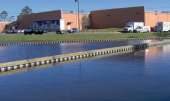
Toewall for Scour Protection
