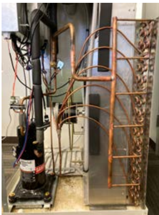
Figure 505 (36k Condensor replacement)
