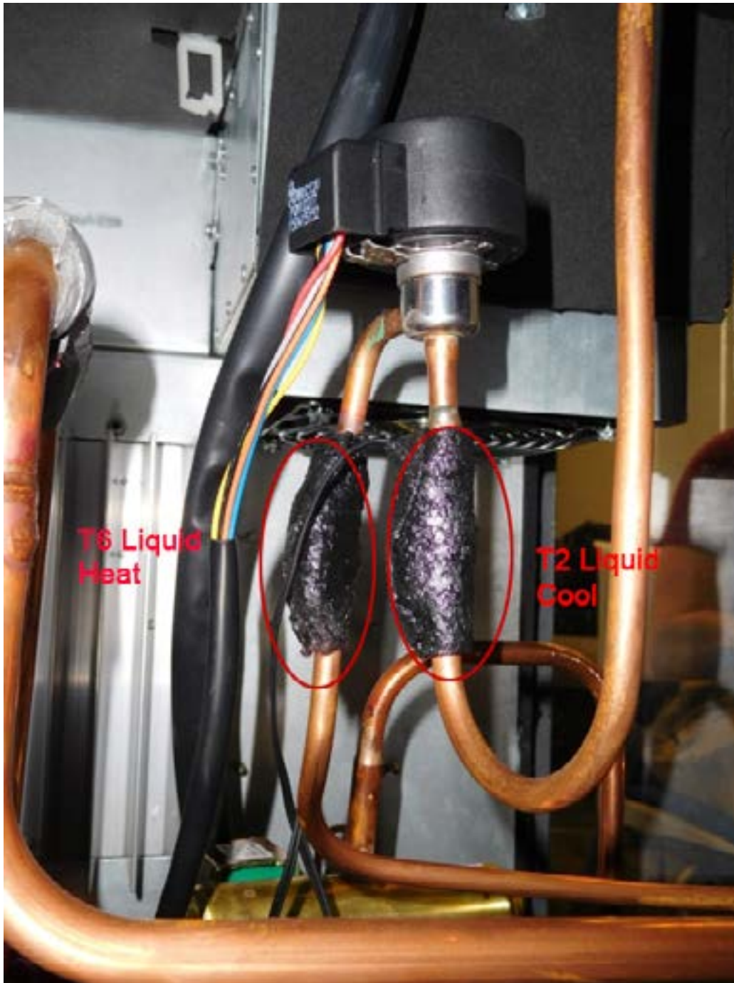
Figure 625 (Thermistor Locations)
