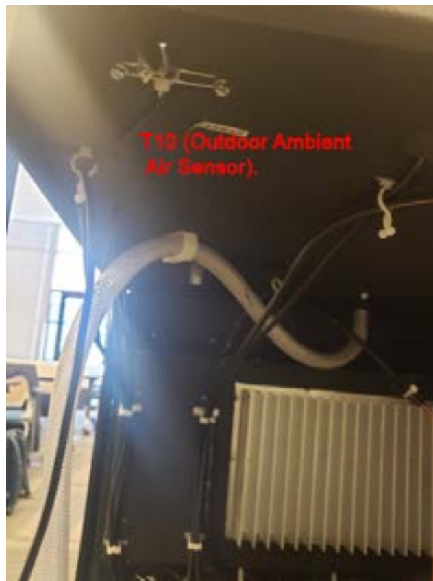
Figure 626 (Thermistor Locations)
