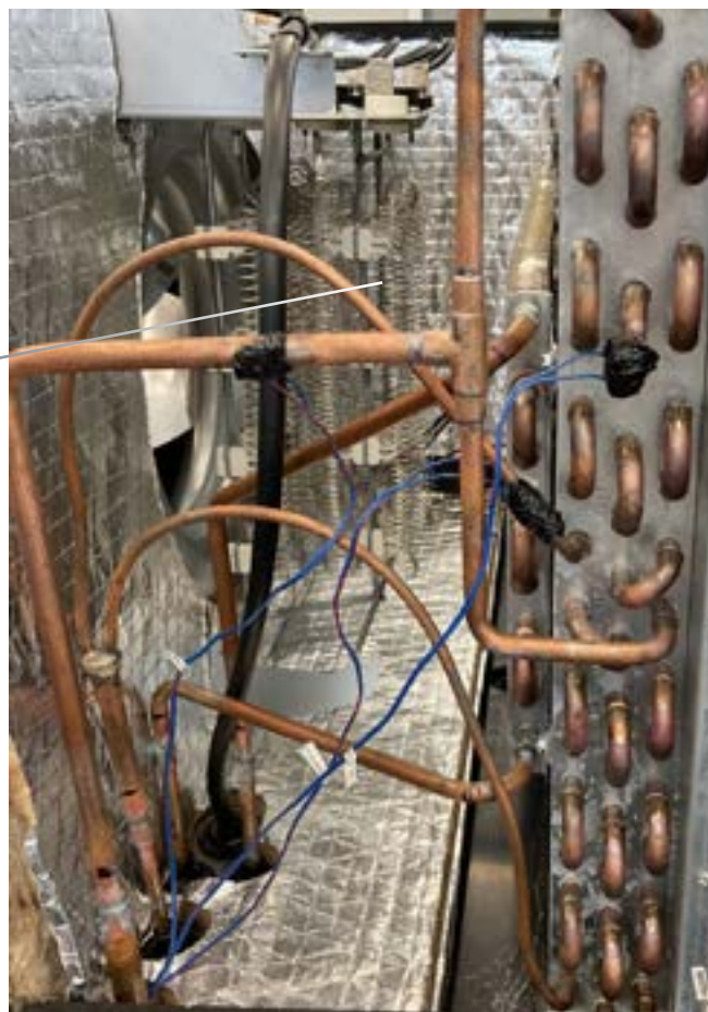
Figure 504 (12k Evaporator coil)
