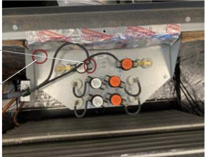
Figure 615 (Heating Elements)
