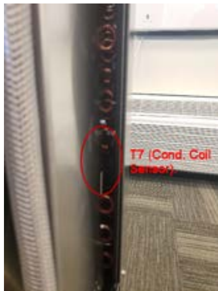
Figure 627 (Thermistor Locations)
