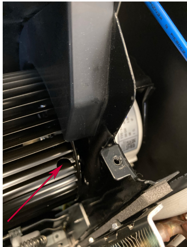
Figure 518 (Blower Wheel Set Screw)
