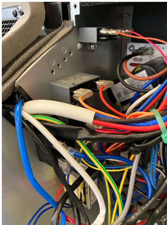
Figure 530 (Disconnect Outdoor Fan Capacitor)
