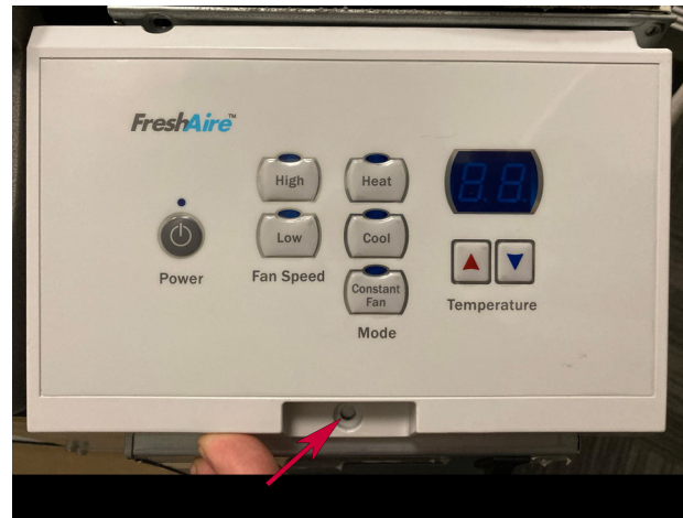
Figure 502 (User Interface Removal)
