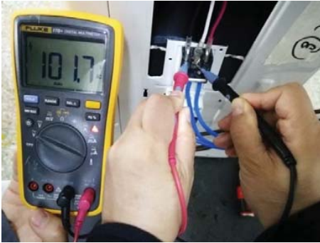
AC voltage test point:
