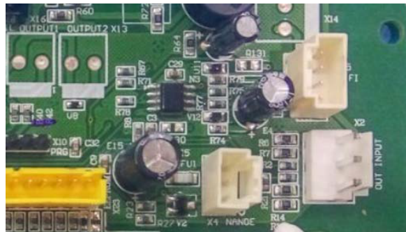
Figure 3 main control board
