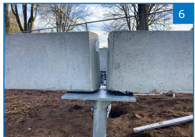
•Completed beam to helical pile connection
