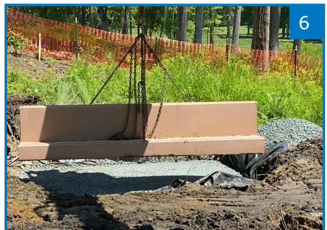
•Abutment handling photo
